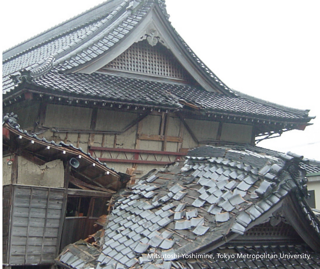
Temple collapse caused by the 2004 Mid Niigata Prefecture Earthquake in Japan
